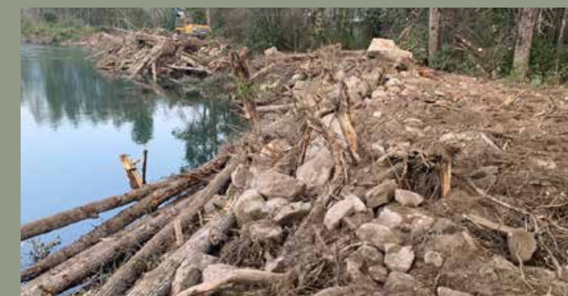
During bank stabilization
