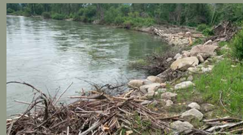
After bank stabilization as high water recedes in June 2023
